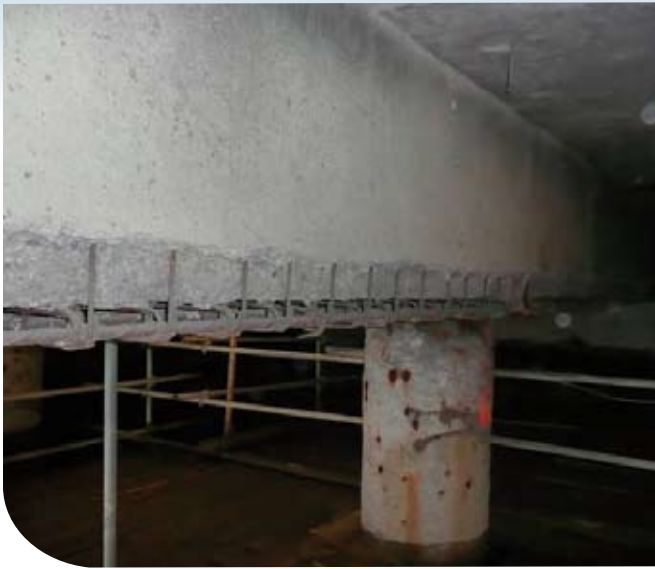
Pilot worksite: a beam before and after repair with wet mix shotcrete
