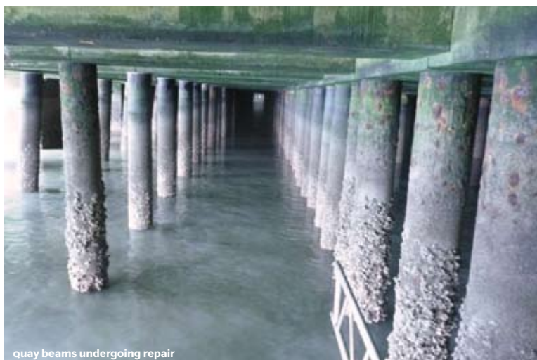
quay beams undergoing repair
